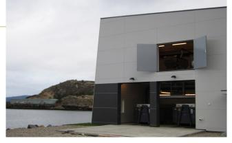
Haus Treatment plant, Norway Built in 2015. Dimensioned for 2500 PE (population equivalent) Maximal waste water flow 37l/s Dimensioned waste water flow 18l/s
